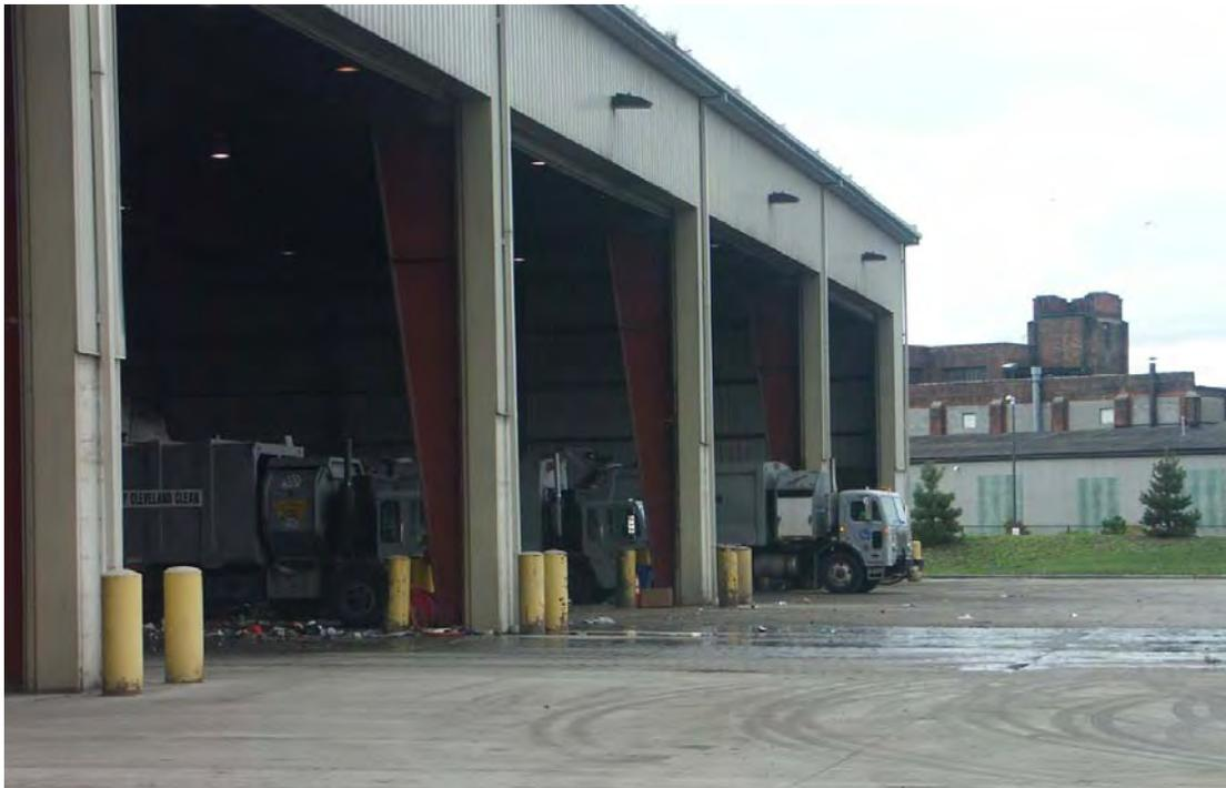
Figure 3. Three-Sided, Trash-Transfer Facility With Bay Doors
