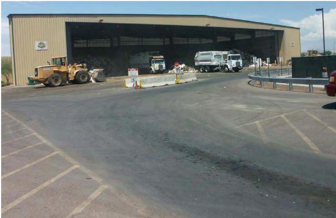
Figure 2. Three-Sided, Open Trash-Transfer Facility
