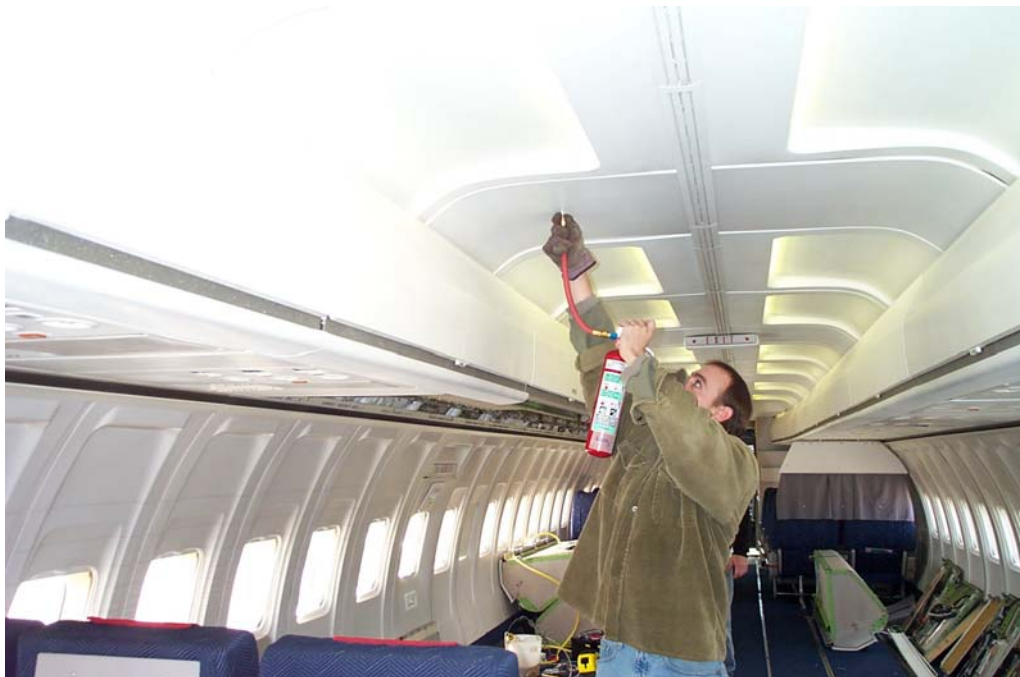
Figure 21. Halon 1211 Discharged Through Ceiling-Mounted Port
