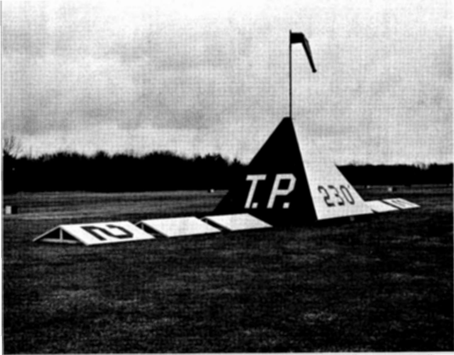
FIGURE 2. LOCATOR PYRAMID WITH R/W ALIGNMENT MARKERS
