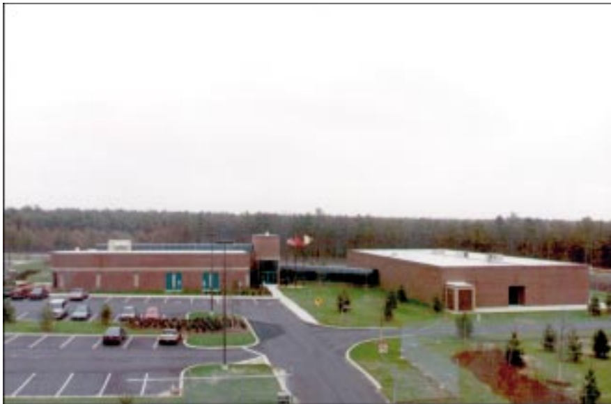
The FAA's Aviation Security Research and Development facility, at the William J. Hughes Technical Center, includes laboratories used for certifying InVision's EDS.
